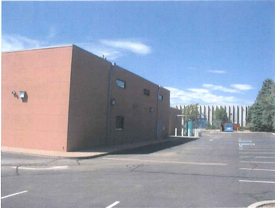
SUBJECT PROPERTY, REAR VIEW, LOOKING NORTH
