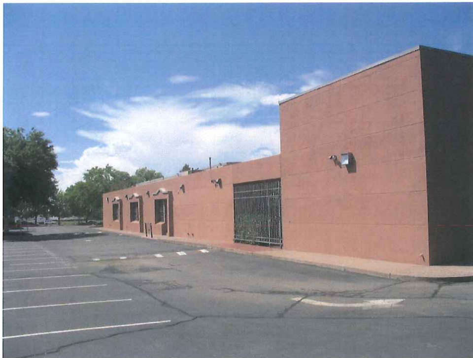
SUBJECT PROPERTY, SOUTH SIDE OF BUILDING, VIEW TO THE NORTHWEST
