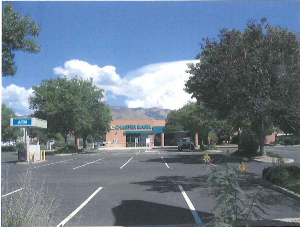
FRONT OF SUBJECT PROPERTY, 2130 EUBANK BLVD NE, VIEW TO THE EAST
