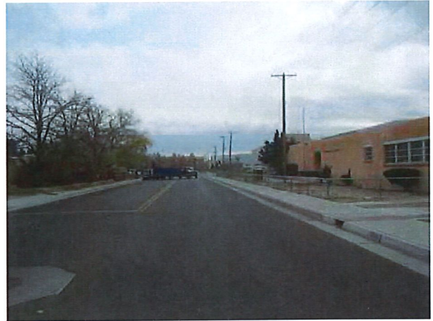
Stanford Drive Looking South
