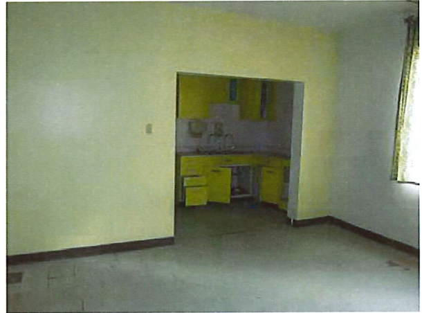
Interior of North Building
