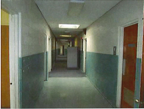
Interior of North Building
