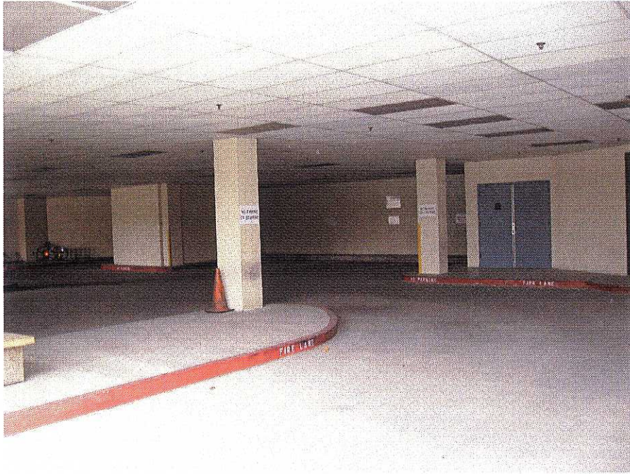
Basement parking area
