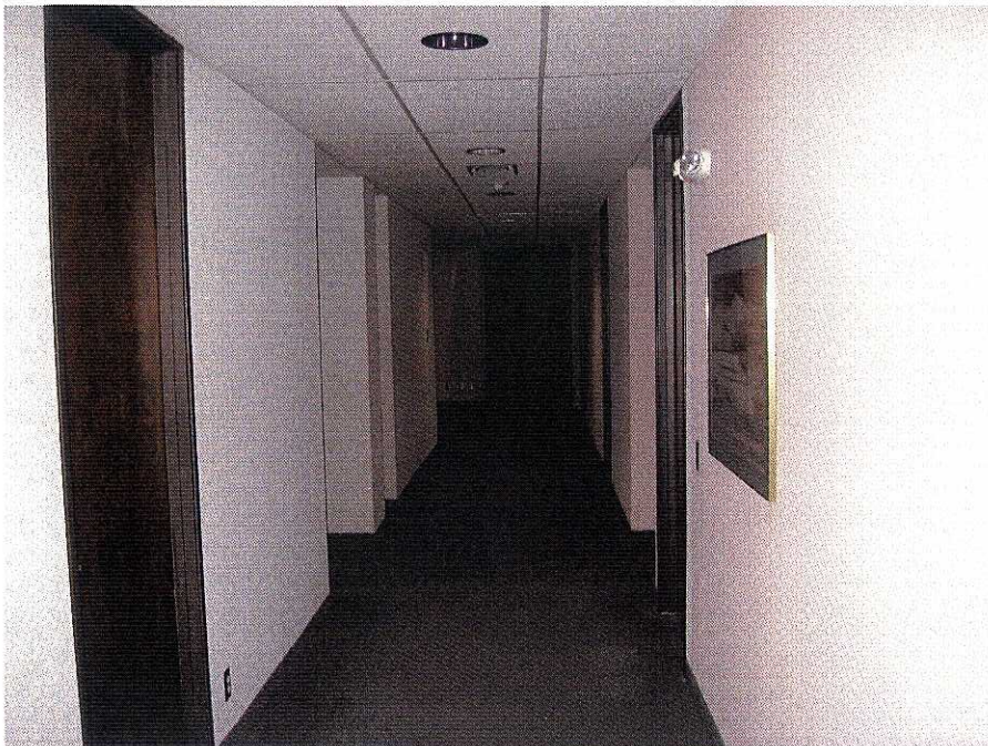
Typical office corridor
