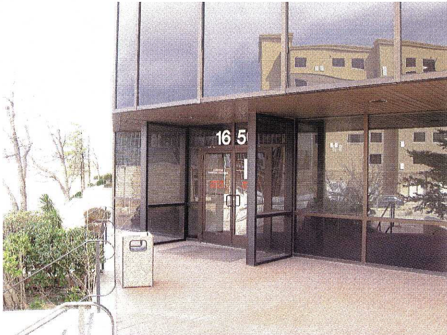
South building entrance
