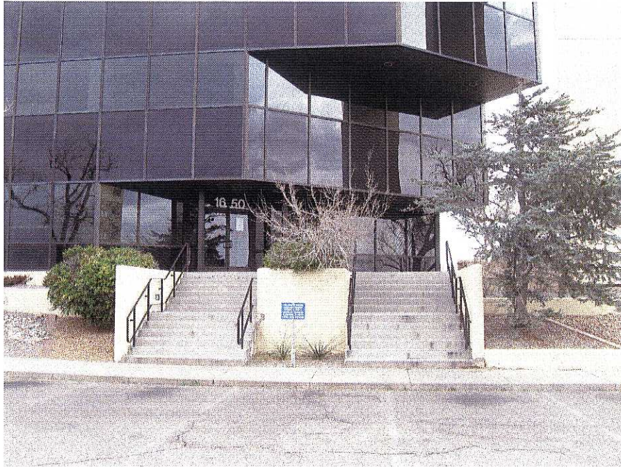
South building entrance
