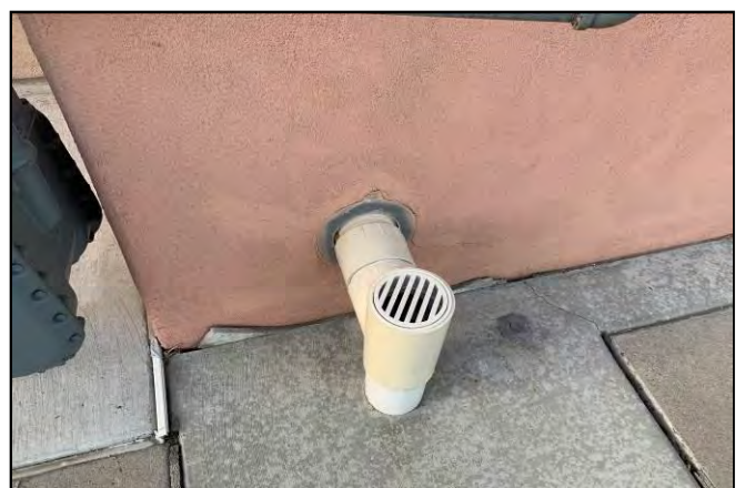
Picture 18 – Roof drain on the exterior of the building.
