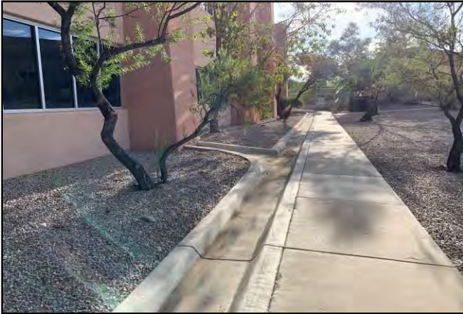
Picture 19 – Roof drains and associated concrete scuppers on the southern portion of the Property.
