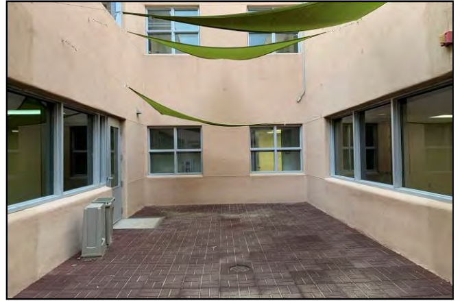
Picture 14 – One of the courtyards and floor drains within the building.
