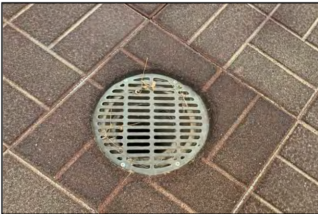
Picture 15 – Closer view of the floor drain within the courtyard.
