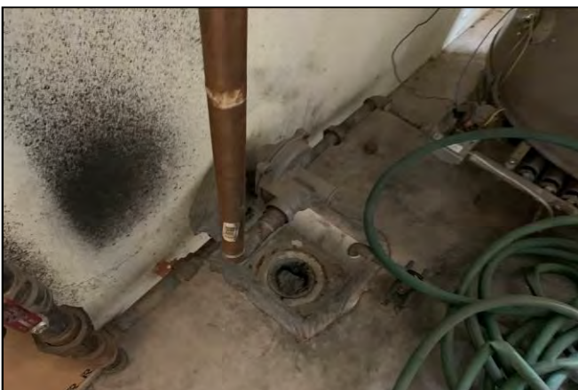
Picture 11 – The floor drain in the maintenance room.
