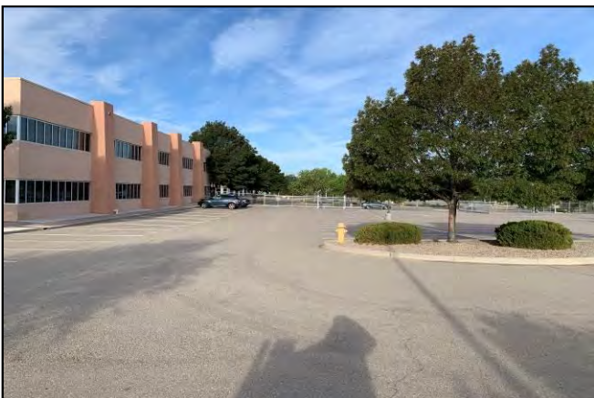
Picture 5 – The parking lot on the northern portion of the Property.
