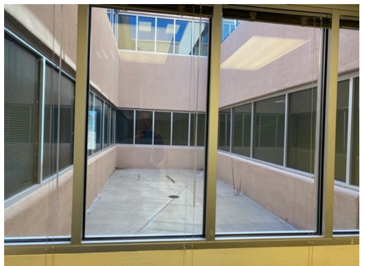
One of four light wells in the central portion of the building.
