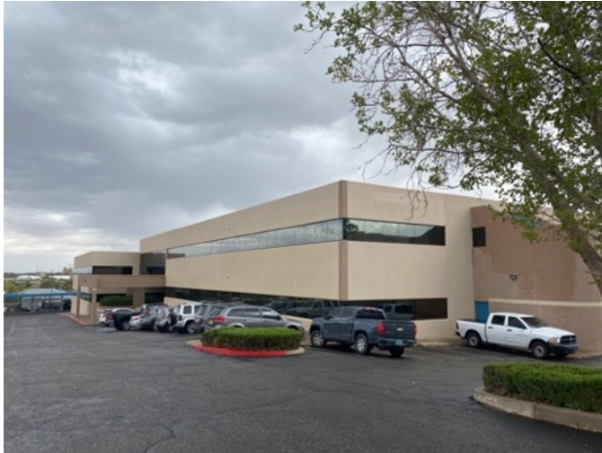
Rental 1: 1601 Randolph Road SE
