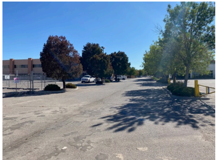
View south on the subject access road with the subject on the left.
