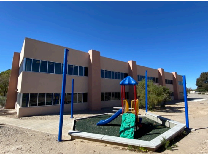
Rear (east) subject building elevation.
