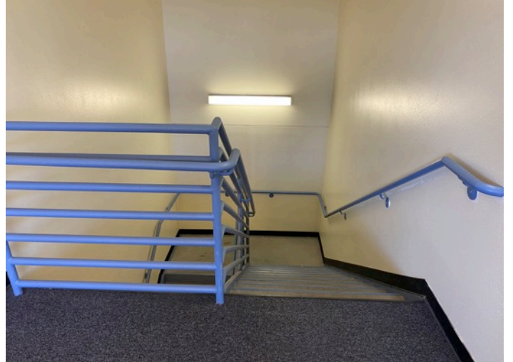
One of two interior stairwells.
