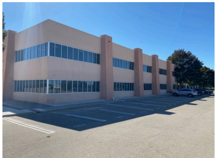
North subject building elevation.
