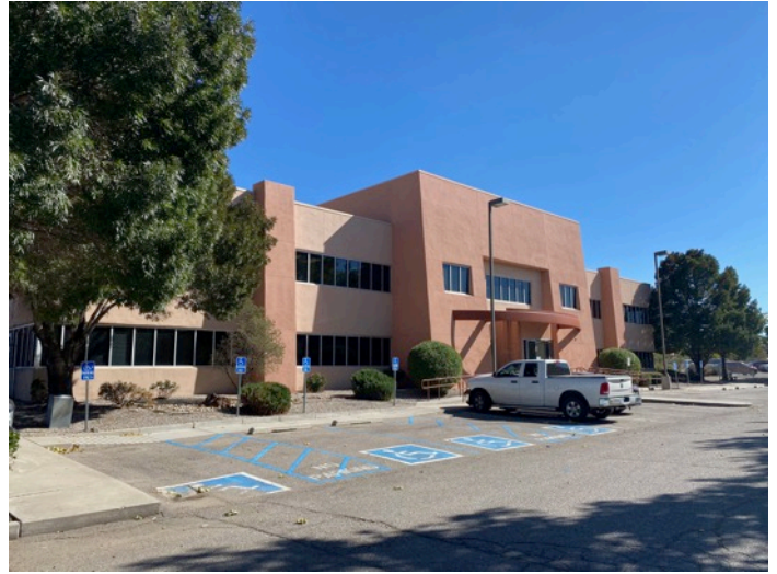
View southeast toward the subject building.
