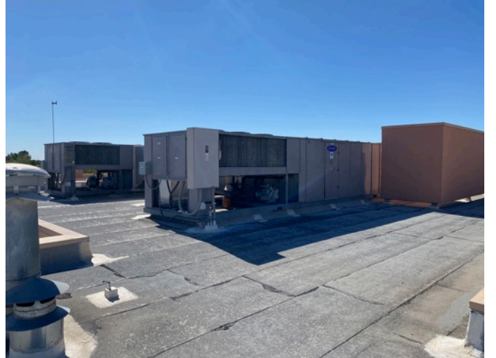
Roof and HVAC units.
