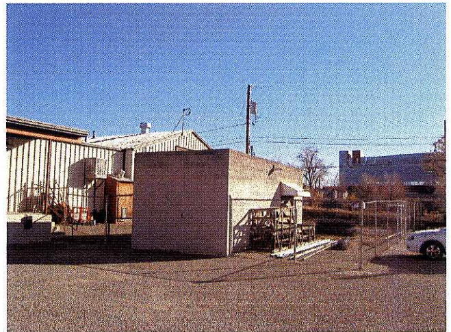
Freestanding storage building
