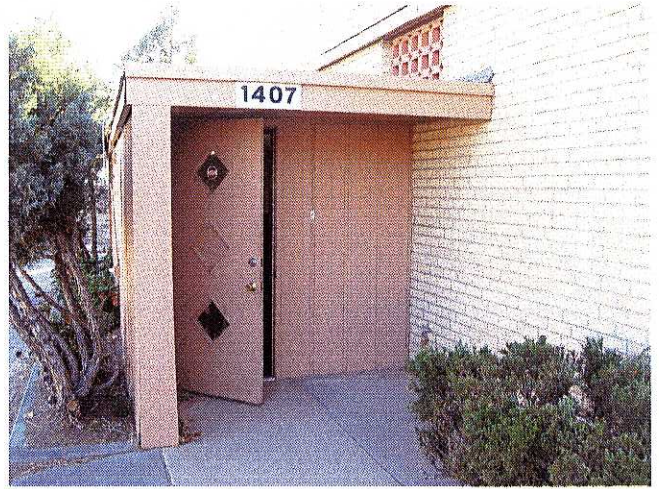
Entrance vestibule to office/showroom area
