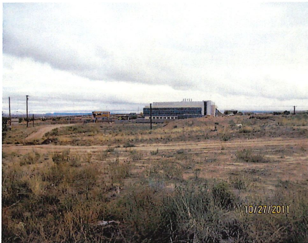
View to the north/northeast taken from the southwest corner of the vacant portion of the site.
