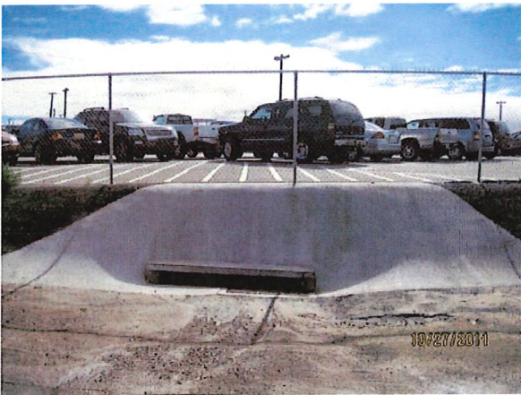
View of the above storm drain from the street.
