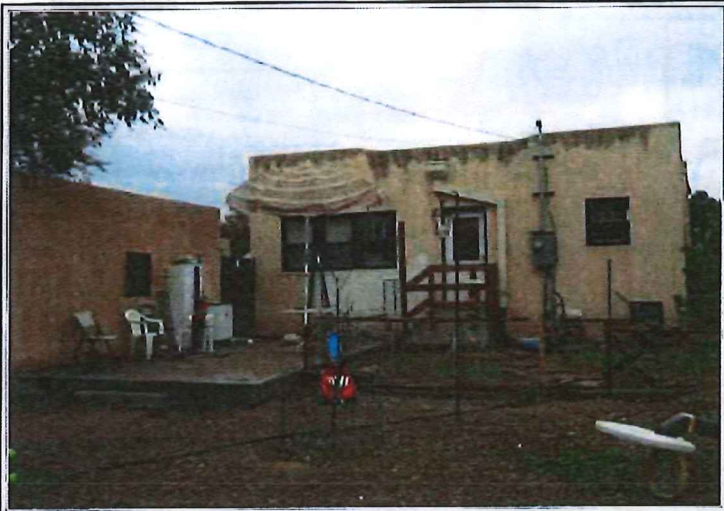
REAR OF SUBJECT PROPERTY
