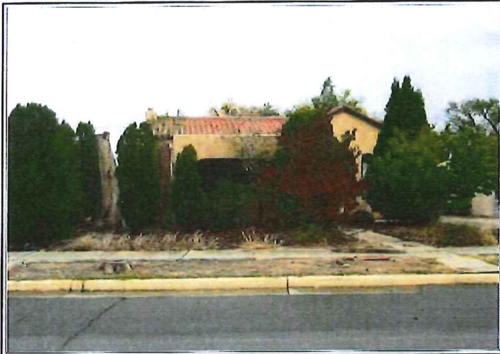
FRONT OF SUBJECT PROPERTY 1709 Las Lomas Rd NE Albuquerque, NM 87106
