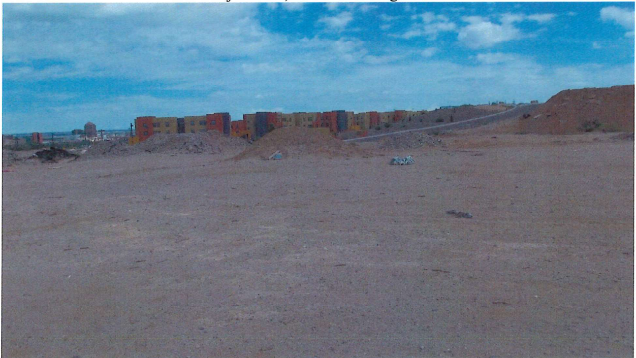
Subject lot 5, block A looking north
