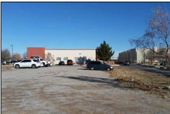
Picture 15 – View of the neighboring commercial/medical facility to the north.
