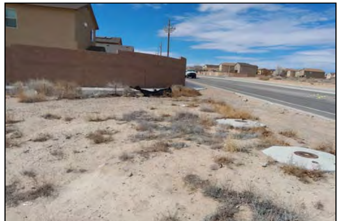
Picture 6 – View of the Property's northwest corner including two water mains, sidewalk, and silt fencing.
